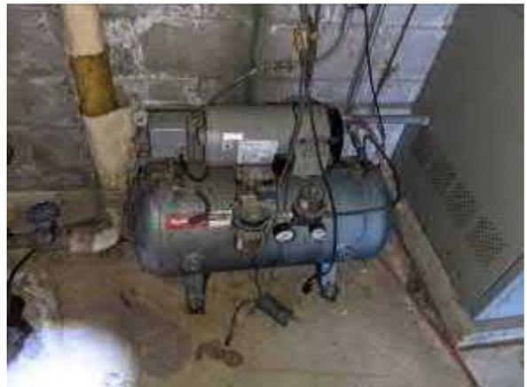
**Photo #58** View of air compressor in mechanical room.
