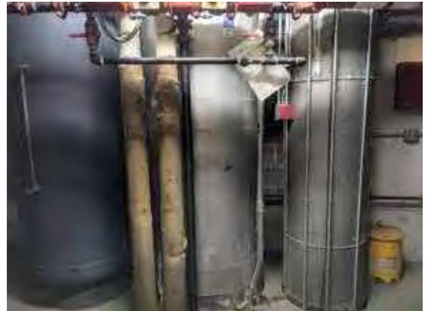
**Photo #8** View of chimneys for boiler system.
