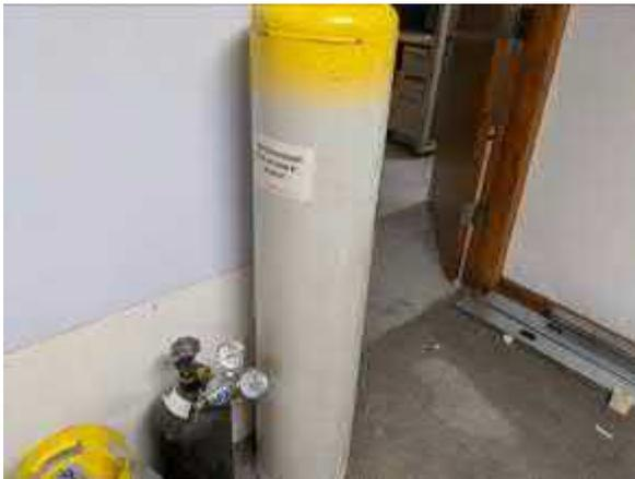
**Photo #39** View of recovered refrigerate tank.
