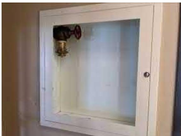
**Photo #11** View of hook-up for fire suppression system, located on each floor.
