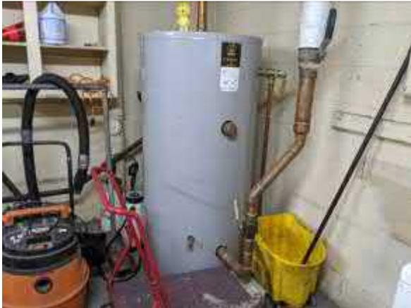
**Photo #33** View of natural gas water heater in laundry area.
