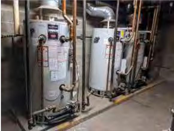
**Photo #25** View of natural gas water heaters.
