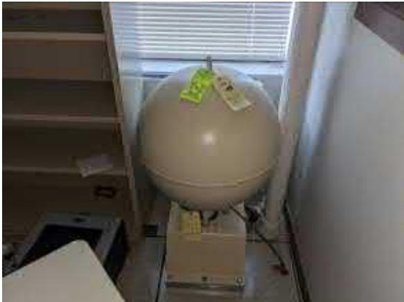
**Photo #63** View of equipment for fire suppression system.
