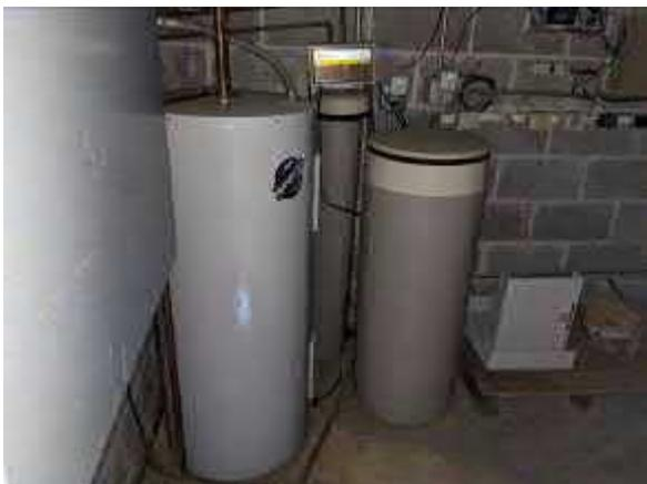
**Photo #59** View of water softener system in mechanical room.
