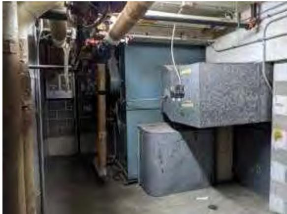
**Photo #7** View of COIL system for heating and cooling system.
