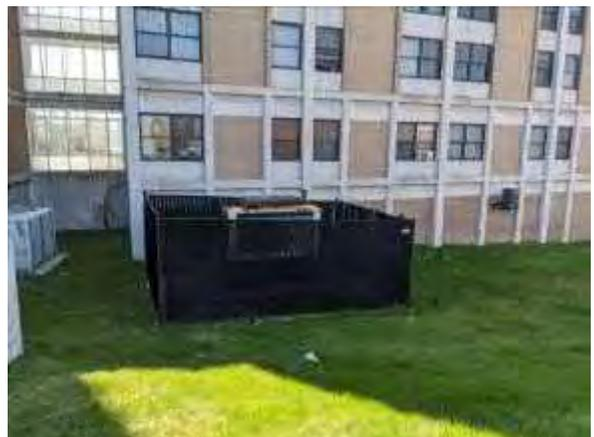
**Photo #66** View of diesel emergency generator on northside of apartment building. View from the north toward the south.
