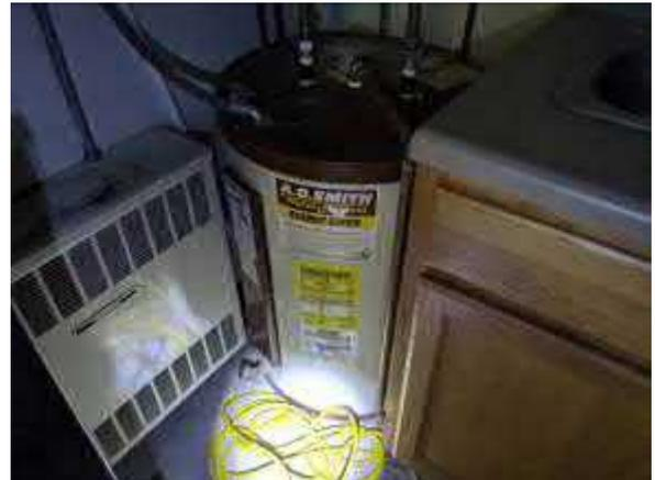
**Photo #52** View of natural gas water heater.
