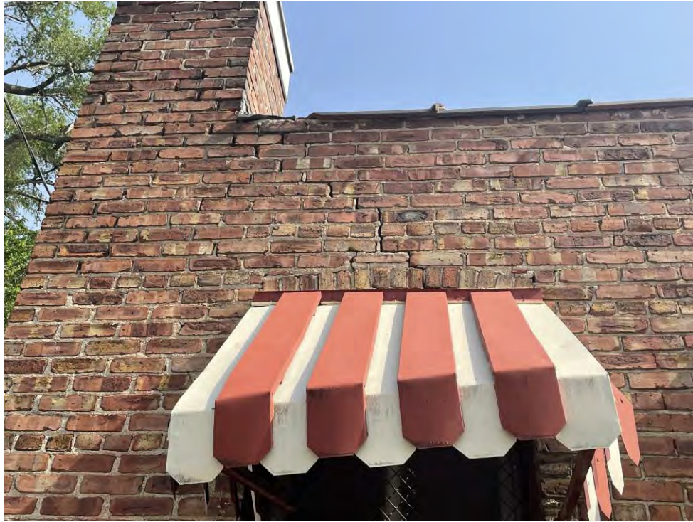
Photo 7. Broken clay roof cap has caused stair step crack. Repair the clay tile cap and tuckpoint the stair step crack.
