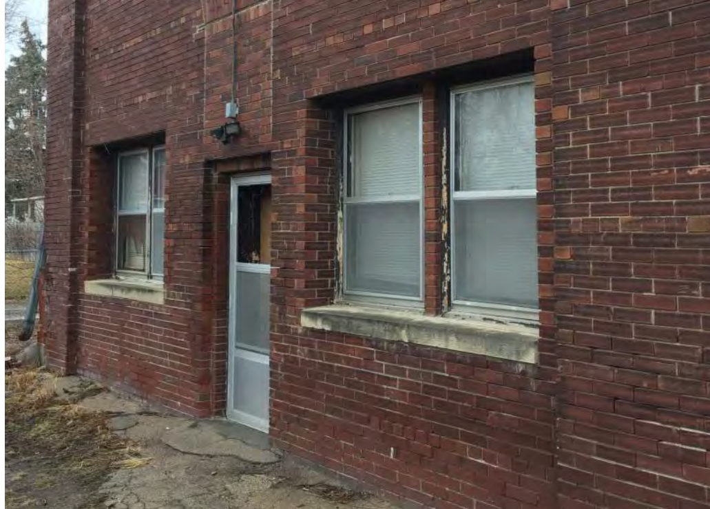
figure A02 - north exterior door
