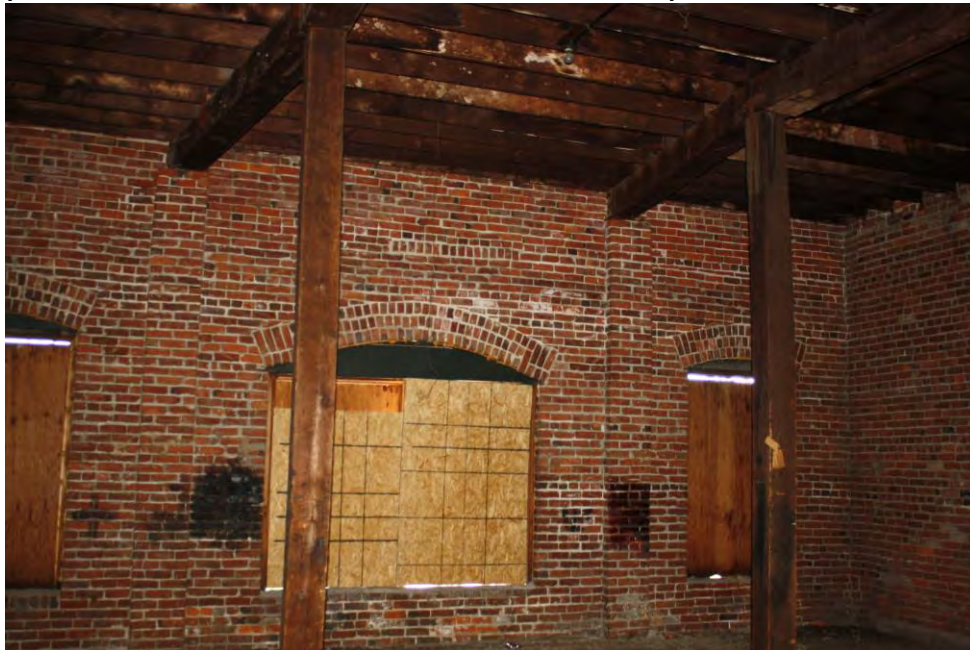
12.3 rd floor, south bay, camera facing east.
