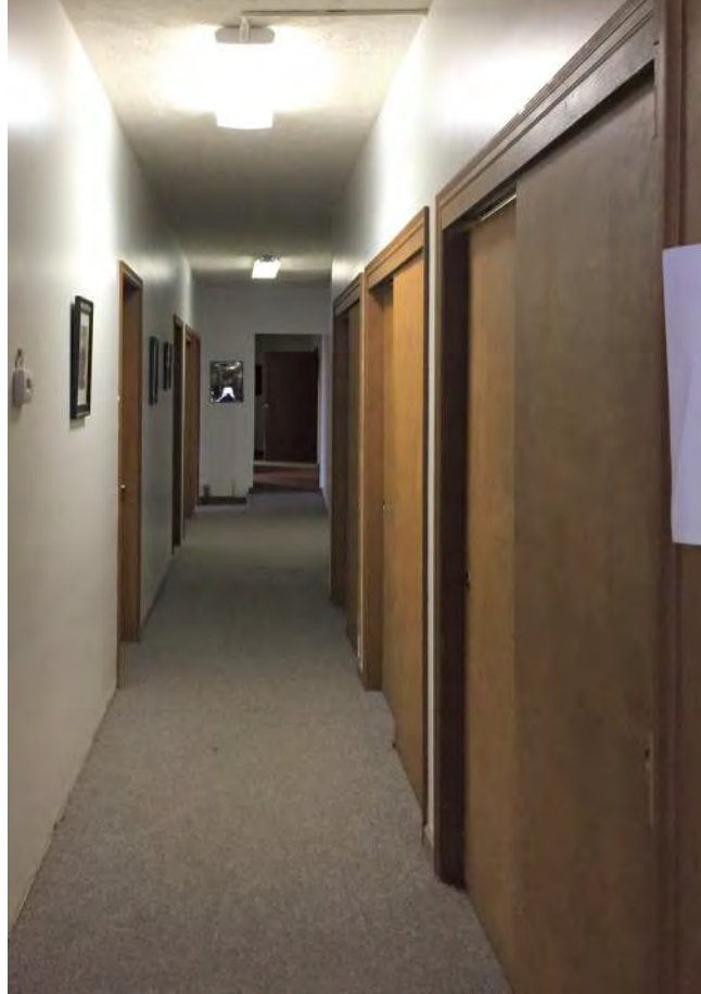
figure A18 - flush wood sliding doors
