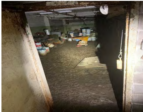
11 Basement of vacant south building.
