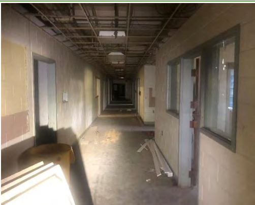
17 View of hallway in vacant north building.
