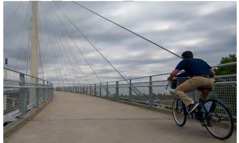
Riding across the Bob Kerrey Bridge. Credit: Chris Orr
