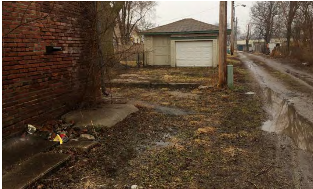
figure L4 north alley looking west
