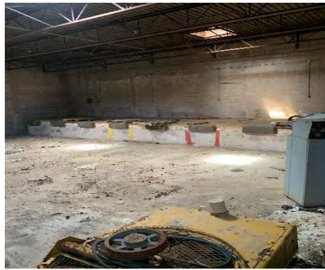
10 Loading dock area in vacant south building.
