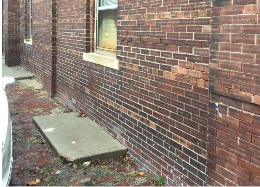
figure A04 - concrete areaway covers at west facade
