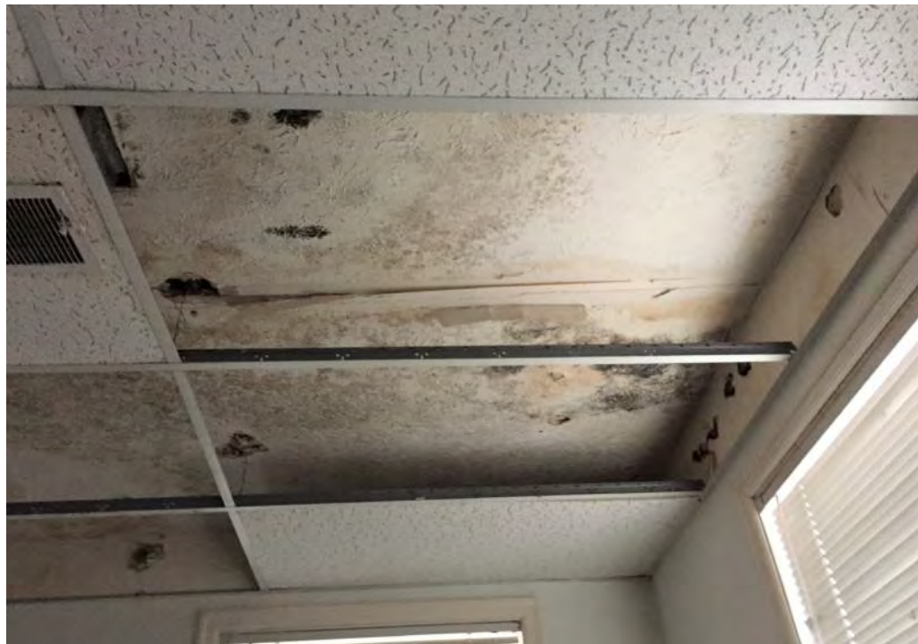
figure A21 - plaster finish above acoustical ceiling
