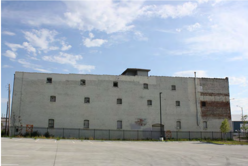
3.South wall, camera facing north.
