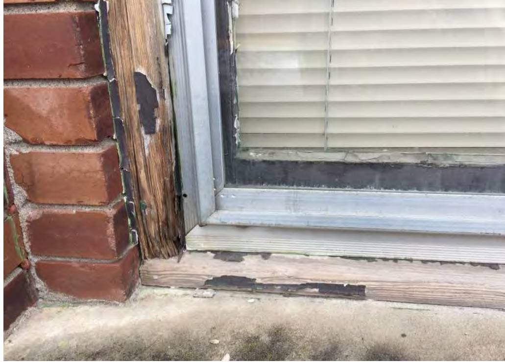
figure A16 - typical wood window with aluminum storm window
