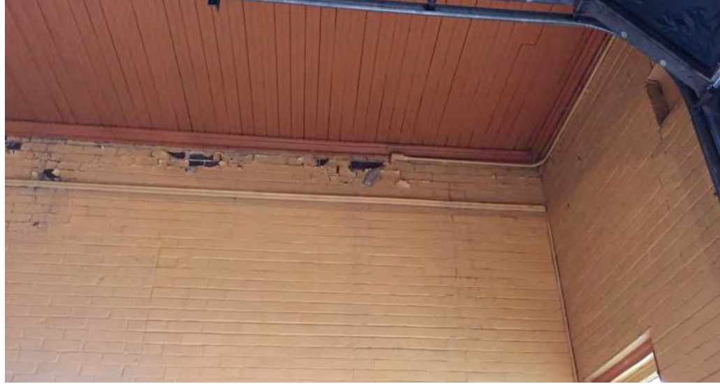
figure A20 - historic bead board ceiling and interior painted brick
