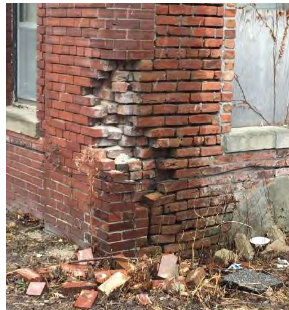
figure S1B - base of northeast corner
