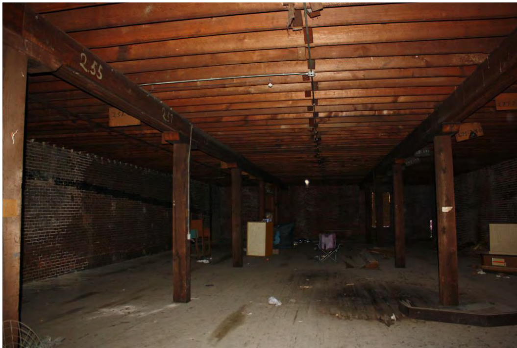
9.2 nd floor, north bay, camera facing west.
