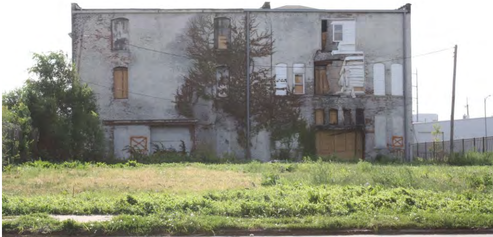
5. West wall, camera facing east.
