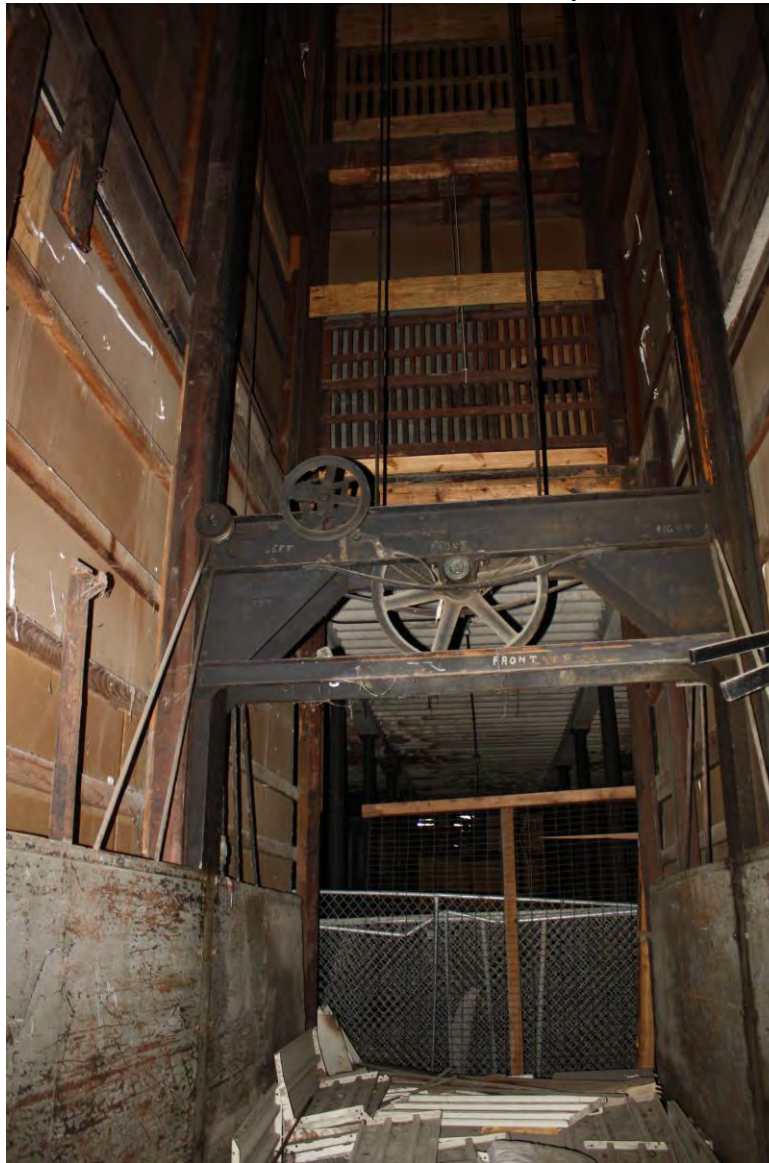
7.Freight elevator in south bay, camera facing west.
