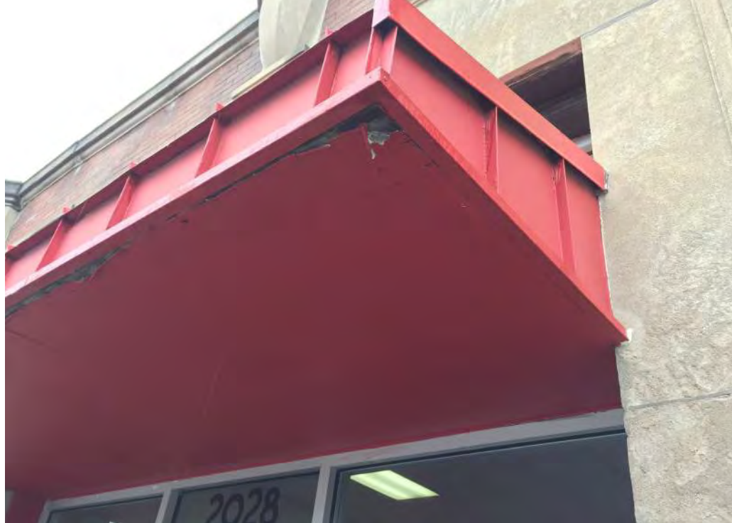
figure A24 - bottom of entrance canopy
