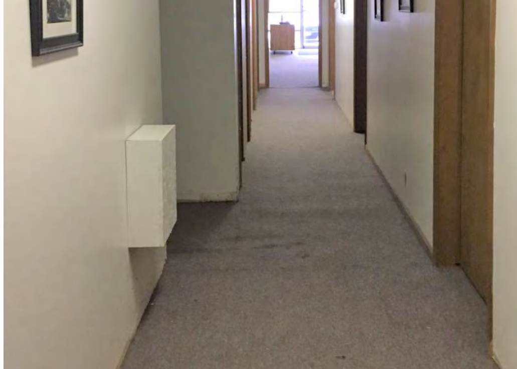
figure A28 - wall box in north corridor
