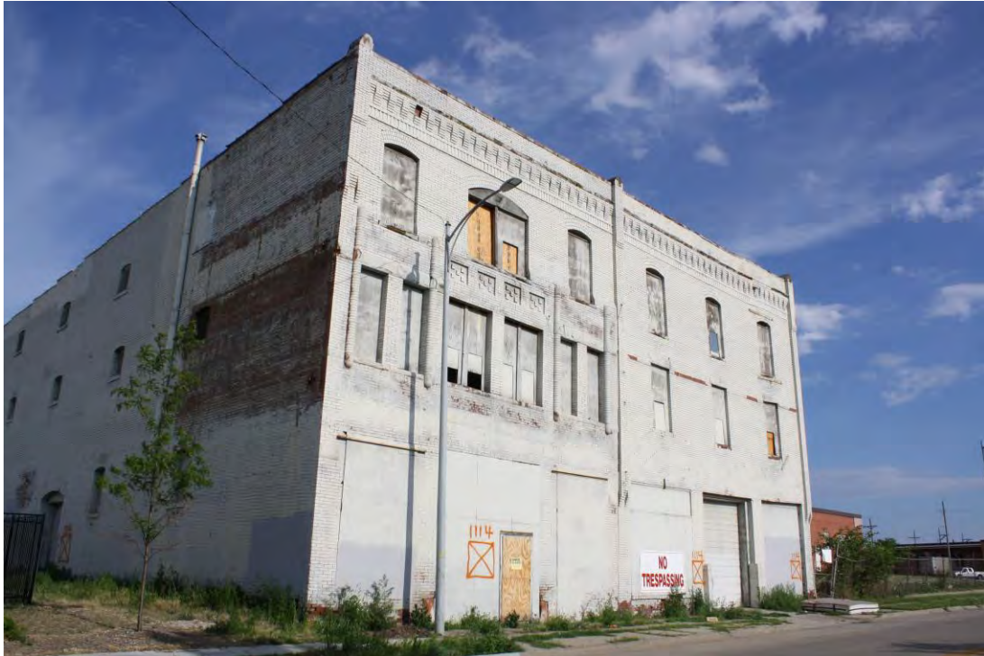
1. Main (east) façade camera looking northwest from Florence Boulevard.
