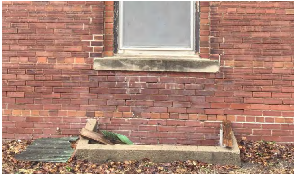
figure A05 - open areaway or window well at east facade
