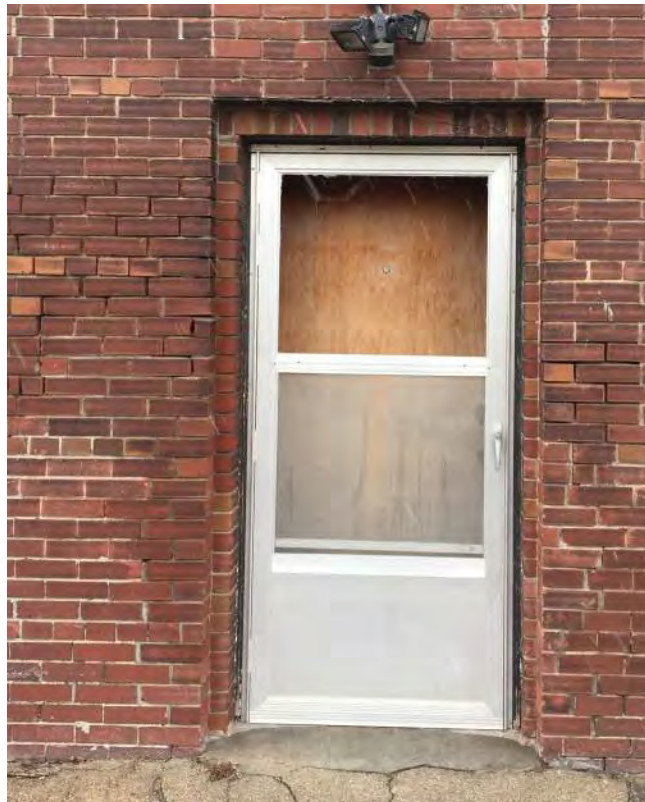
figure A15 - exterior door, west facade
