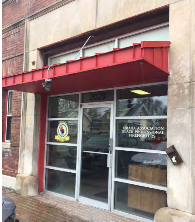
figure A14 - aluminum storefront entrance
