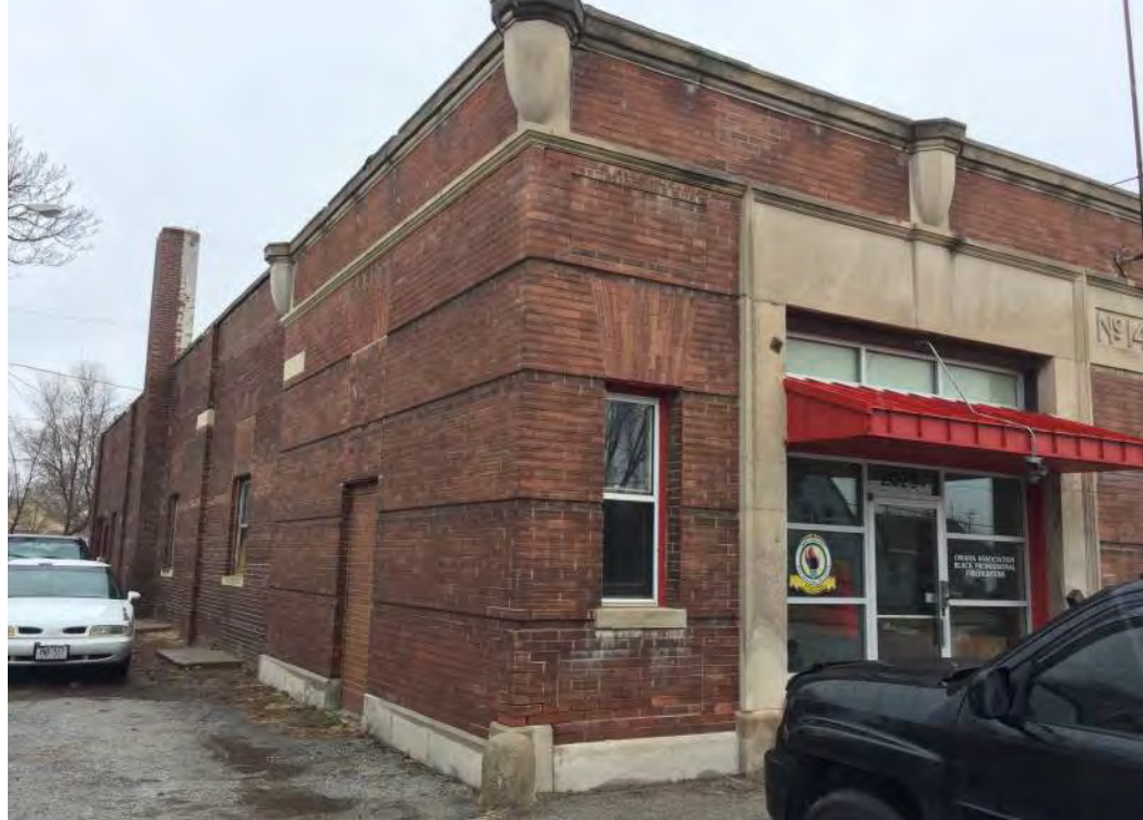
figure A08 - typical stone masonry at exterior
