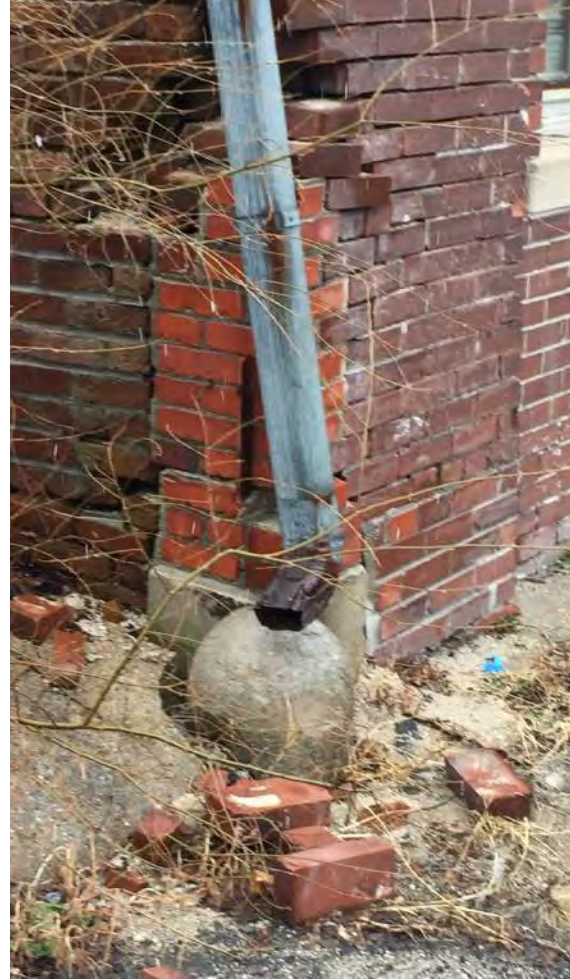
figure S2AB - base of northwest corner
