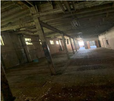
1 Interior view of vacant south building.
