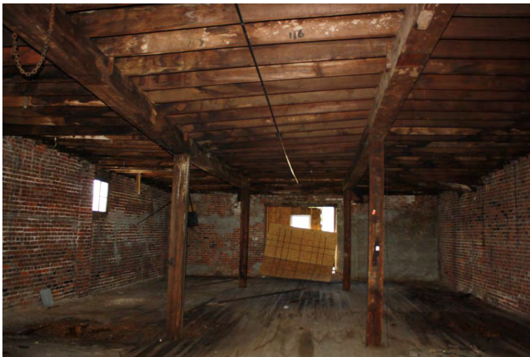
11. 3 rd floor, south bay, camera facing west.
