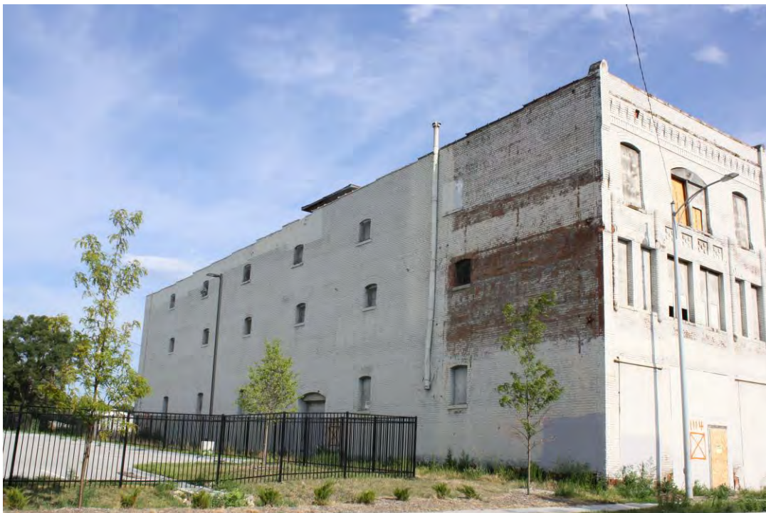
2. South wall, camera looking northwest.
