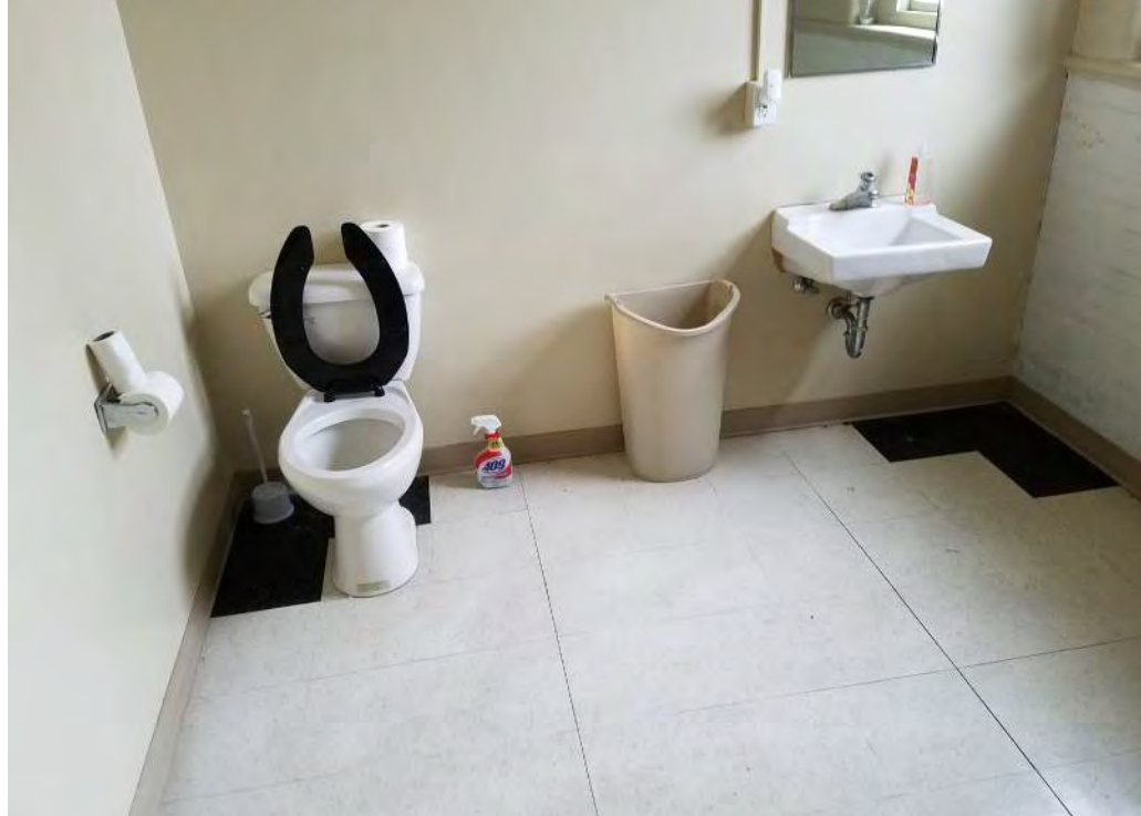
figure M2 - women's restroom plumbing fixtures
