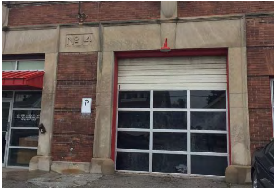
figure A13 - aluminum overhead door at southeast bay (garage)
