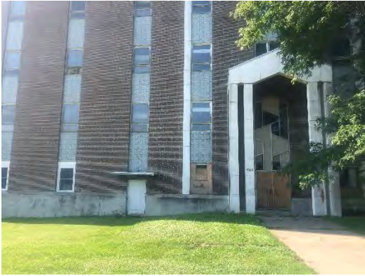
13 View of vacant north building.
