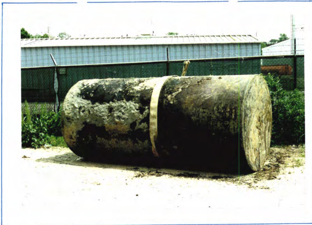
Photo #1. Facing south, the east end of the tank still has a good asphalt coating on it. The west end has almost no coating on it due to past overfills.
