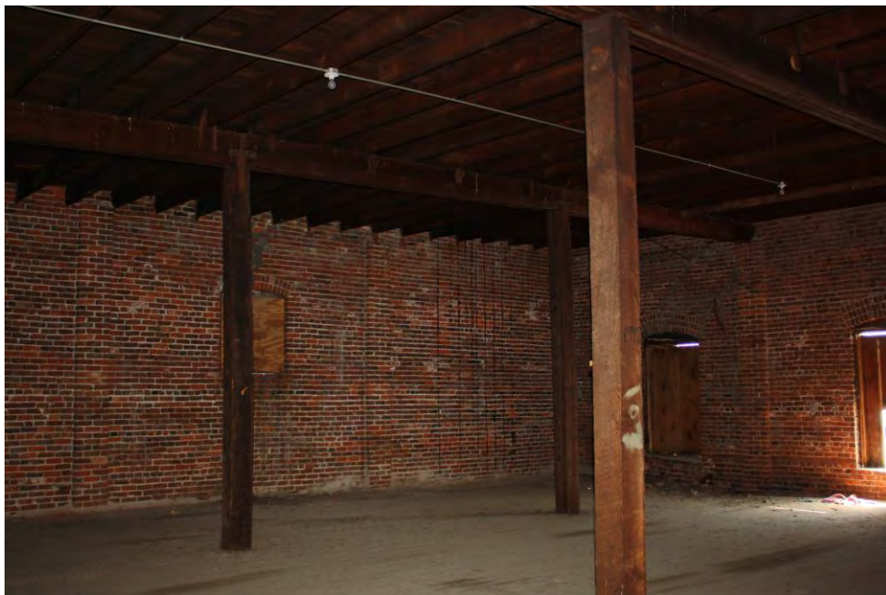
13.3 rd floor, north bay camera facing northeast.
