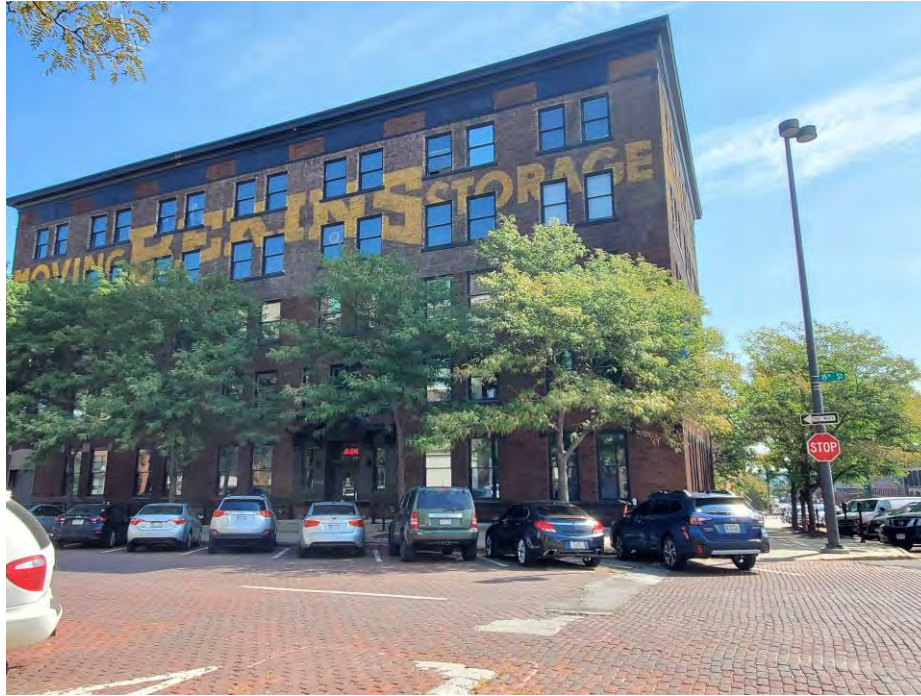
Former Bekins Building at 621 S 15 th Street. This building was built as the Western Newspaper Union in 1916 and later converted to Bekins storage. It has been rehabilitated and today houses apartments. Re-opening previously infilled windows impacted the visibility of the Bekins sign.
