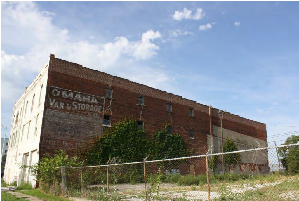
4.North wall, camera facing south.
