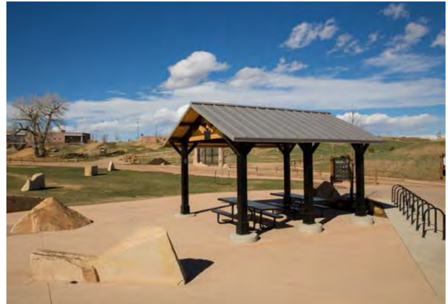
Pavilion and bike racks
