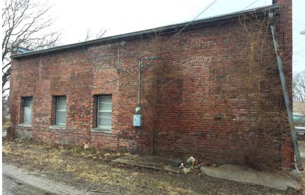
figure A12 - gutter and downspout at north facade
