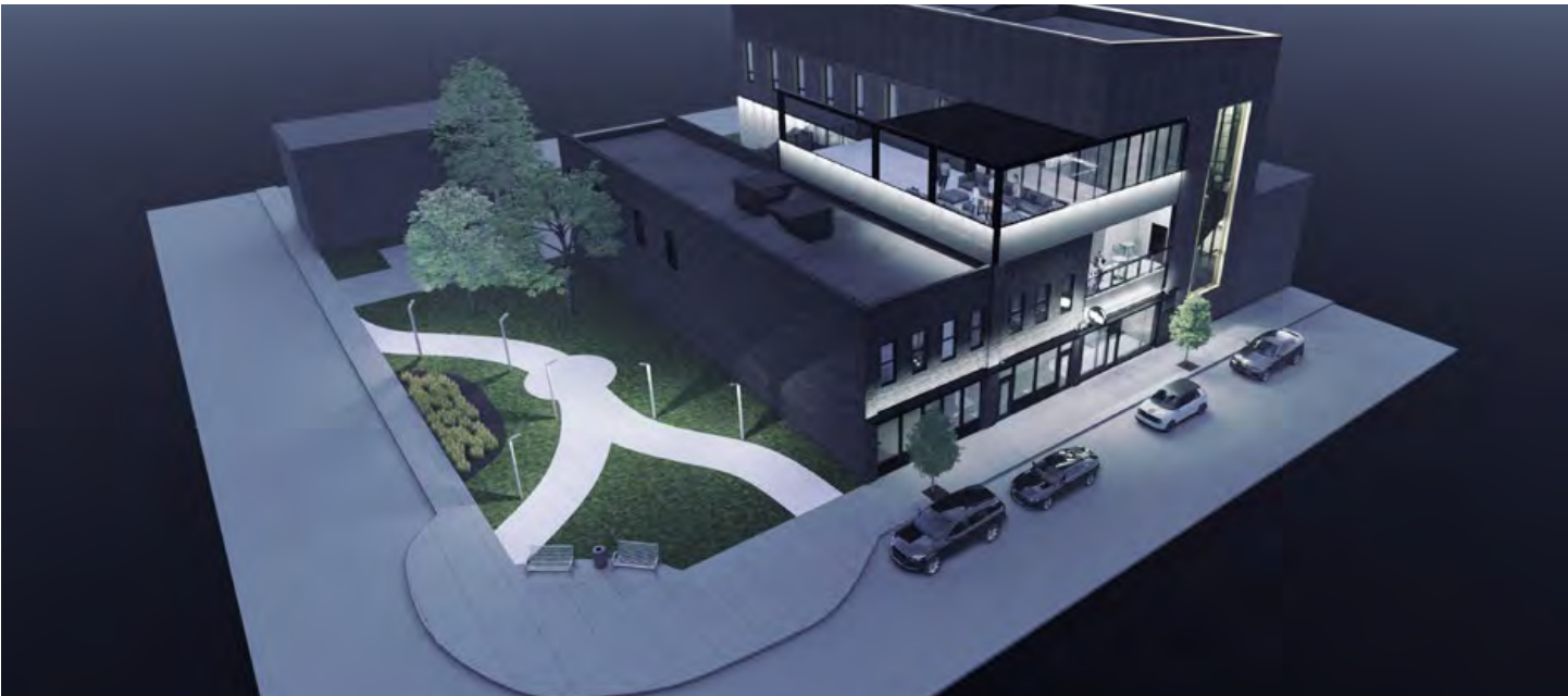
Aerial from corner of 24th and Lake Streets
