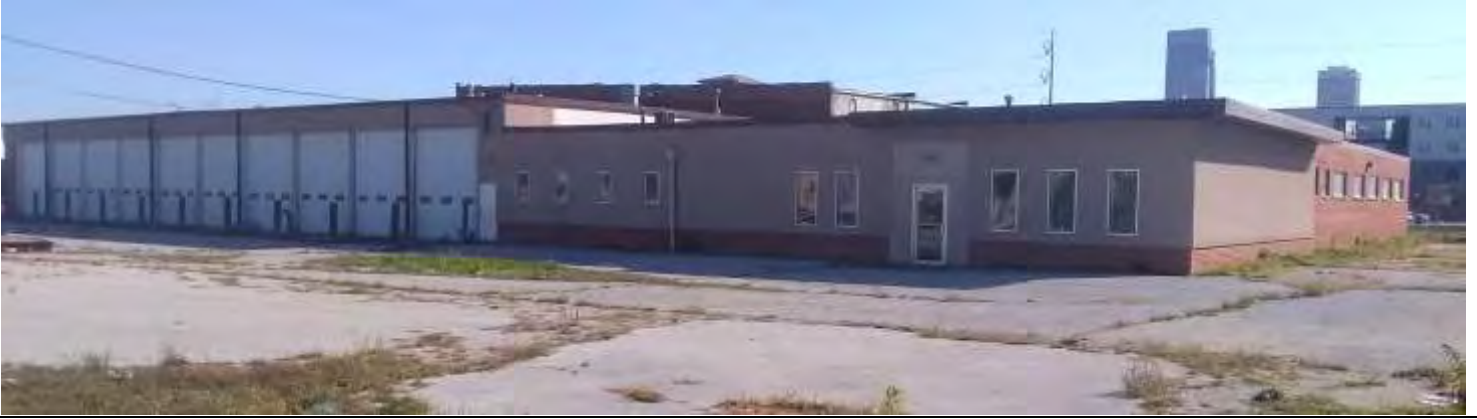
Looking southeast at the north/front and west sides of the Site building.
