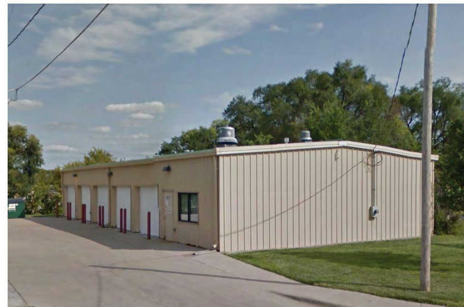
5 5213 S 29 STREET 1 STORY 3 100 SF
