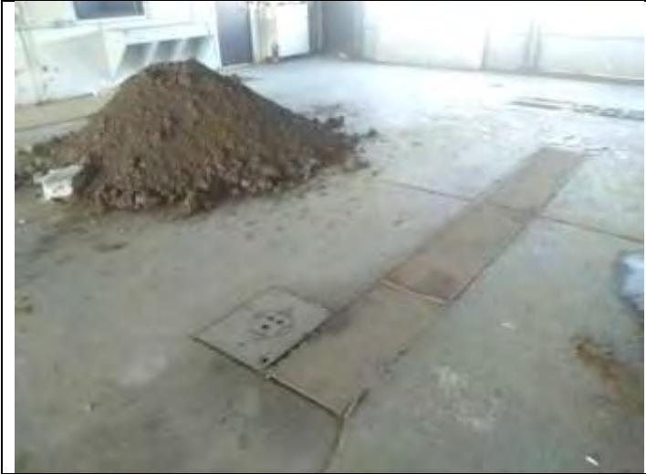
Views of suspected former buried/underground hydraulic vehicle lifts.
