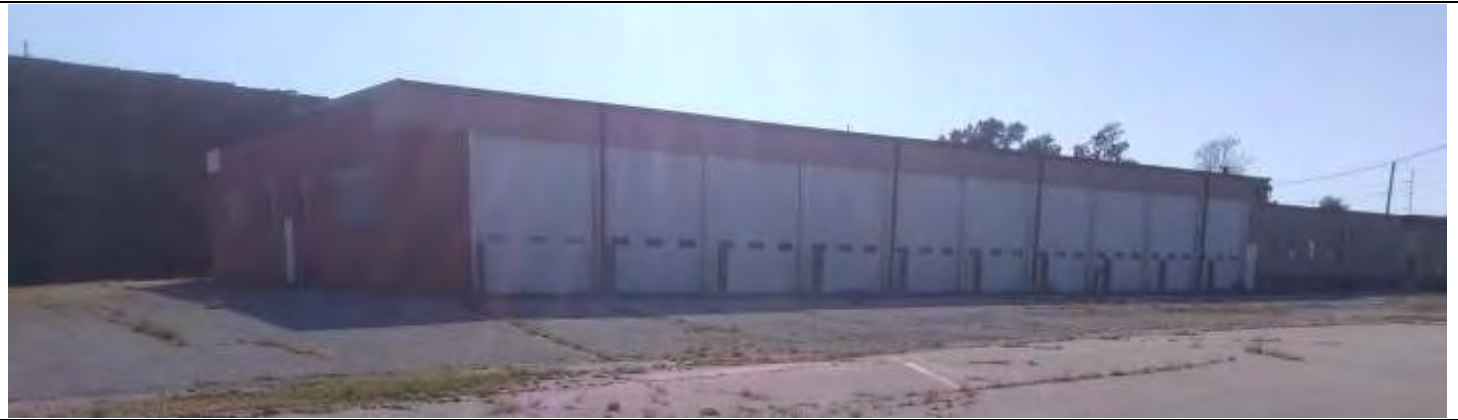
Looking southwest at the east and north/front sides of the Site building.
