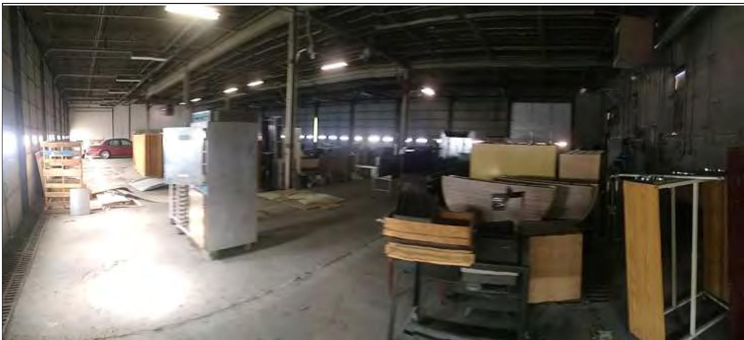
Looking northwest at the main/east side vehicle storage garage bay area.
