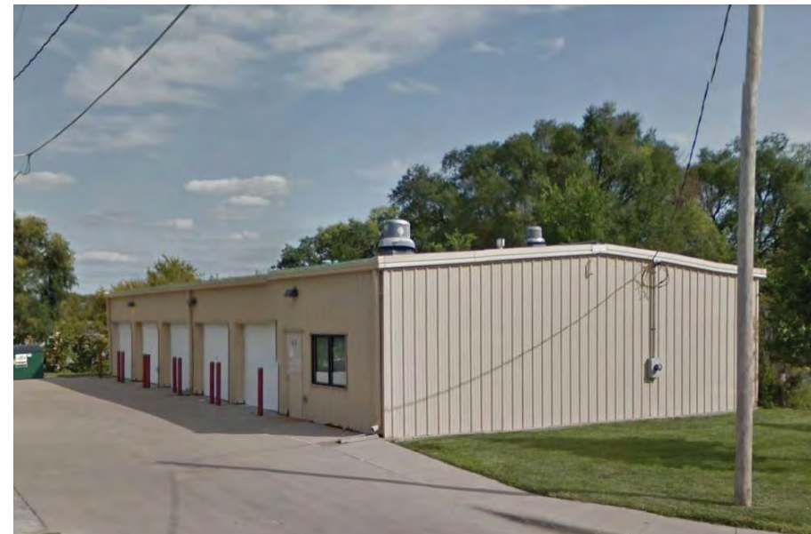
5 5213 S 29 STREET 1 STORY 3 100 SF
