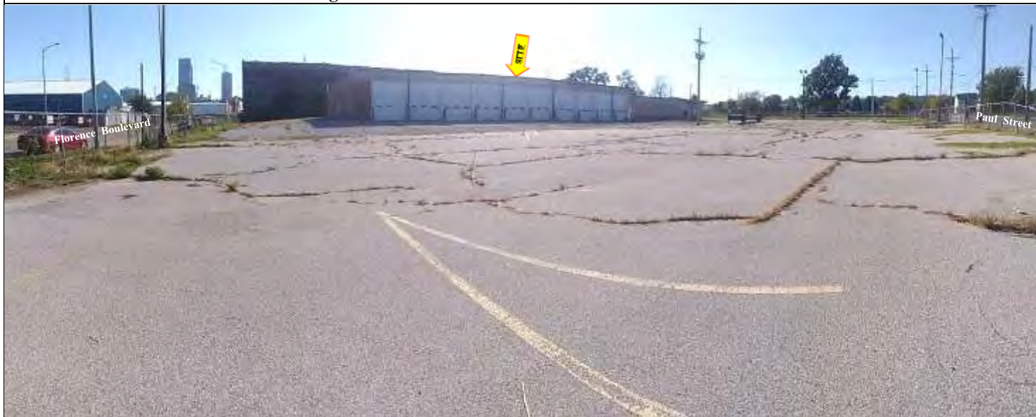
Looking southwest at the east and north/front sides of the Site.
