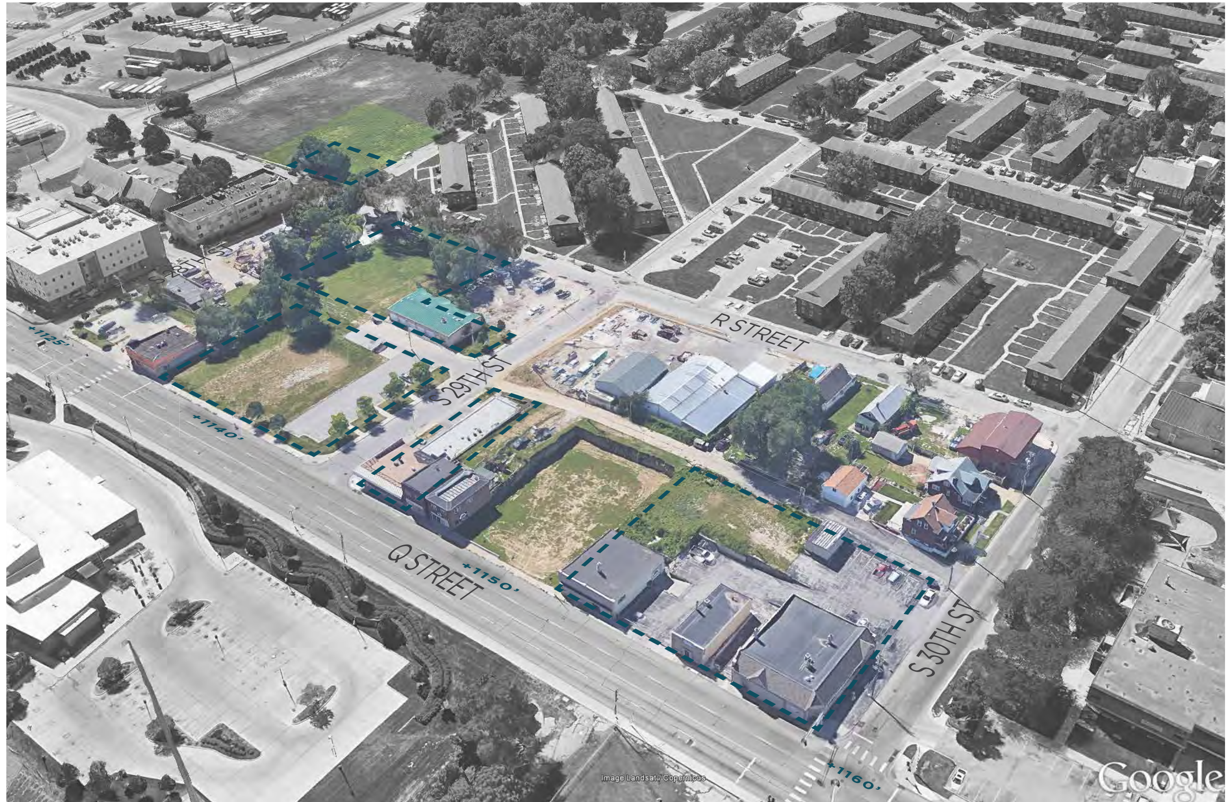
Aerial Site View LOOKING SOUTHEAST
