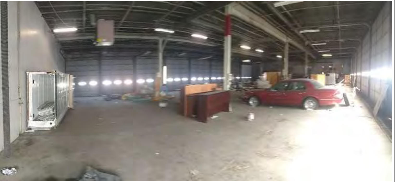
Looking northeast at the main/east side vehicle storage garage bay area.
