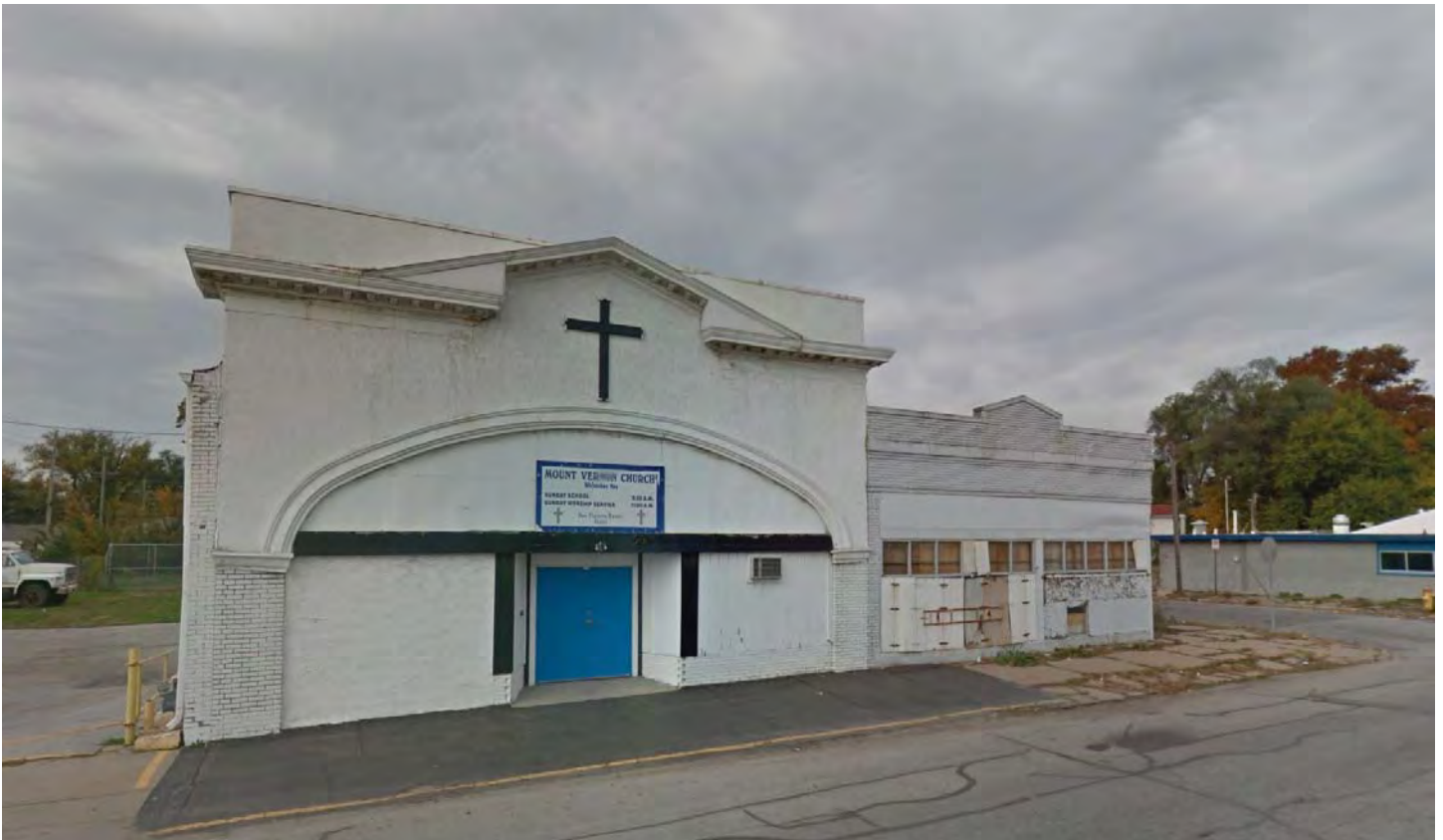
Current View Looking Northwest
