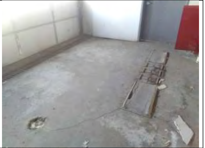
Views of suspected former buried/underground hydraulic vehicle lifts.
