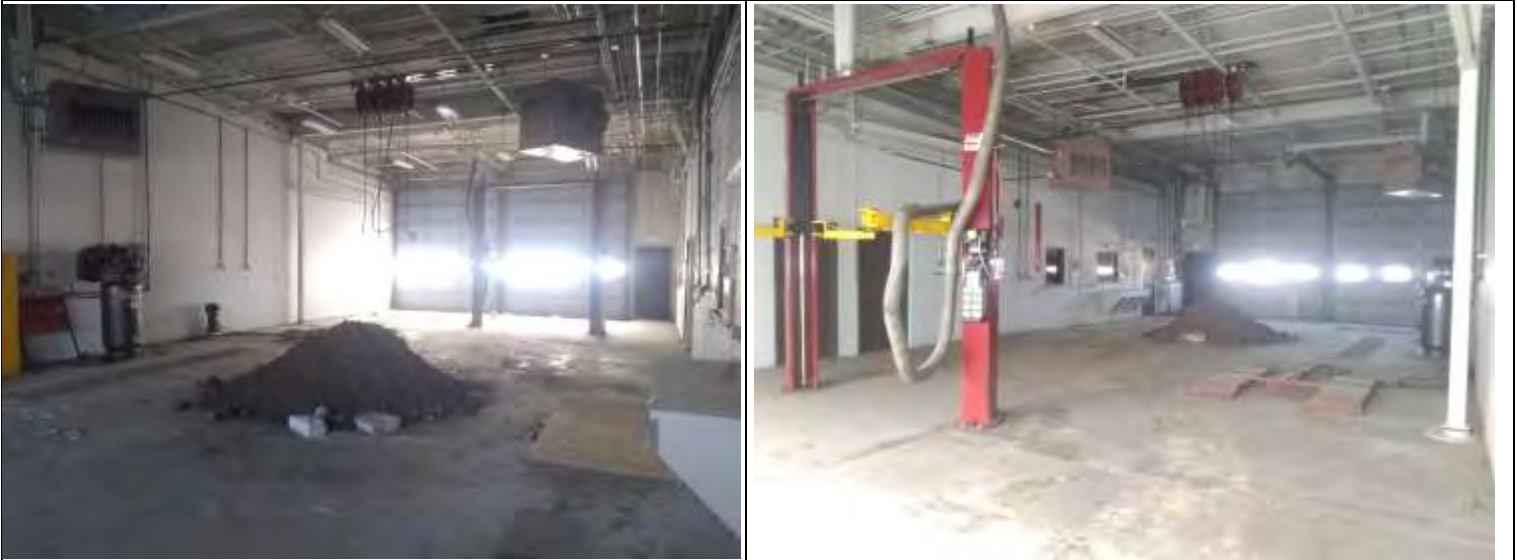
Views of middle vehicle maintenance bay.
