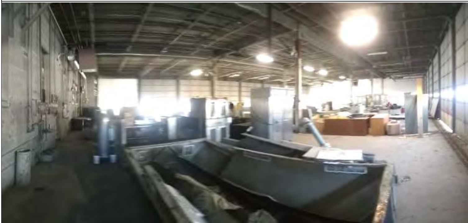
Looking southwest at the main/east side vehicle storage garage bay area.
