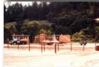
Cornell Bridge Access Site
